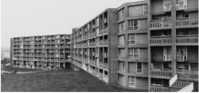
District heating delivers clean from coal
