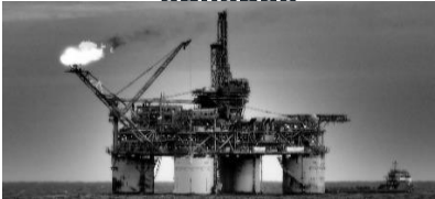
North Sea Gas discovered – UK heat network development stops while European networks advance
