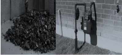
Coal fire heat networks converted to gas
